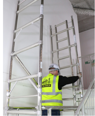
Fit a plain 4 rung frame to the ladder portal frame and engage the interlock clips.
