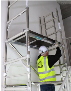
Fit a platform to the 2nd rung of the 4 rung plain frame with the trapdoor on the ladder frame side.
