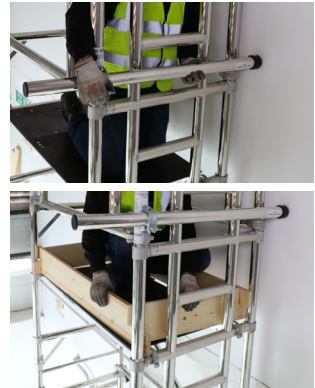
Fit 2 side props every 2m, one either end of the tower. If you cannot fit side props, stabilizers shall be fitted to all 4 corners of the tower. They shall be fitted to create the largest footprint possible. Then fit your toe-boards using the clips.
