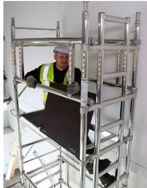
Sitting through the platform, fit 2 guardrail frames, one either side or 4 Horizontal braces 2 either side with hooks facing out. Repeat steps 1 - 5 to build additional heights Ensure hooks are fully engaged.
