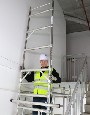
Fit a plain 4 rung frame to the plain portal frame and engage the interlock clips.
